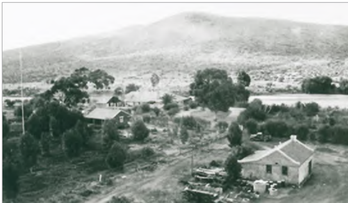
Figure 7. Photograph of Paratoo Homestead 1934 (courtesy of SLSA, B18329/1)
