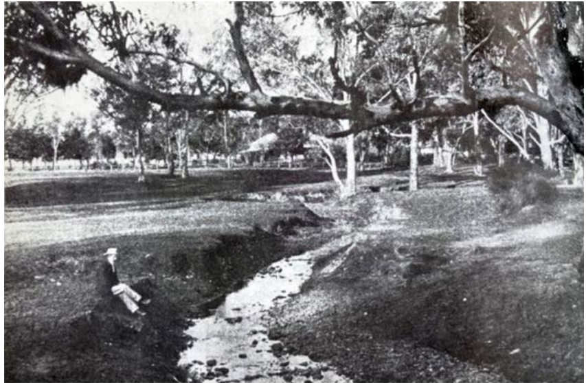
Figure 5 – Second Creek crossing Knightbridge near Rochester Street, Leabrook (from the Critic, December 1903, reproduced in Warburton 1961)
