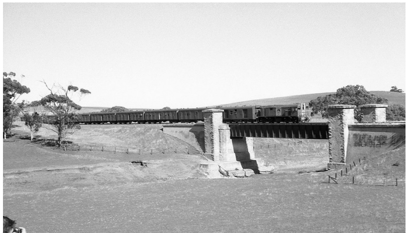
Figure 2. Gouge's bridge over the Light River, south of Kapunda, constructed 1860, photographed May 1989. Image from Tiller (2012).
